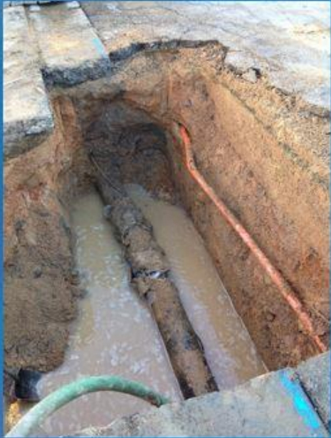
AFR & DOUGLAS – 2016 10-IN STEEL PIPE FAILURE
