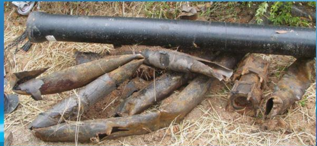
PARK VISTA STEEL MAIN REPLACEMENT - 2009
