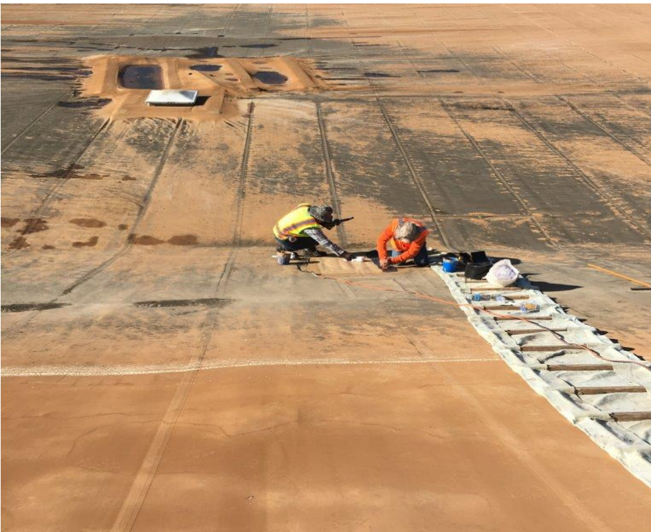
Figure 2. Photo showing extraction/patching of new sample location.
