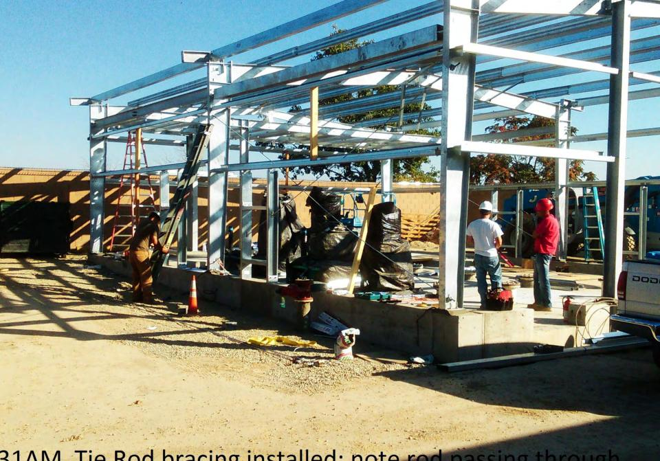
31AM Tie Rod bracing installed; note rod passing through
