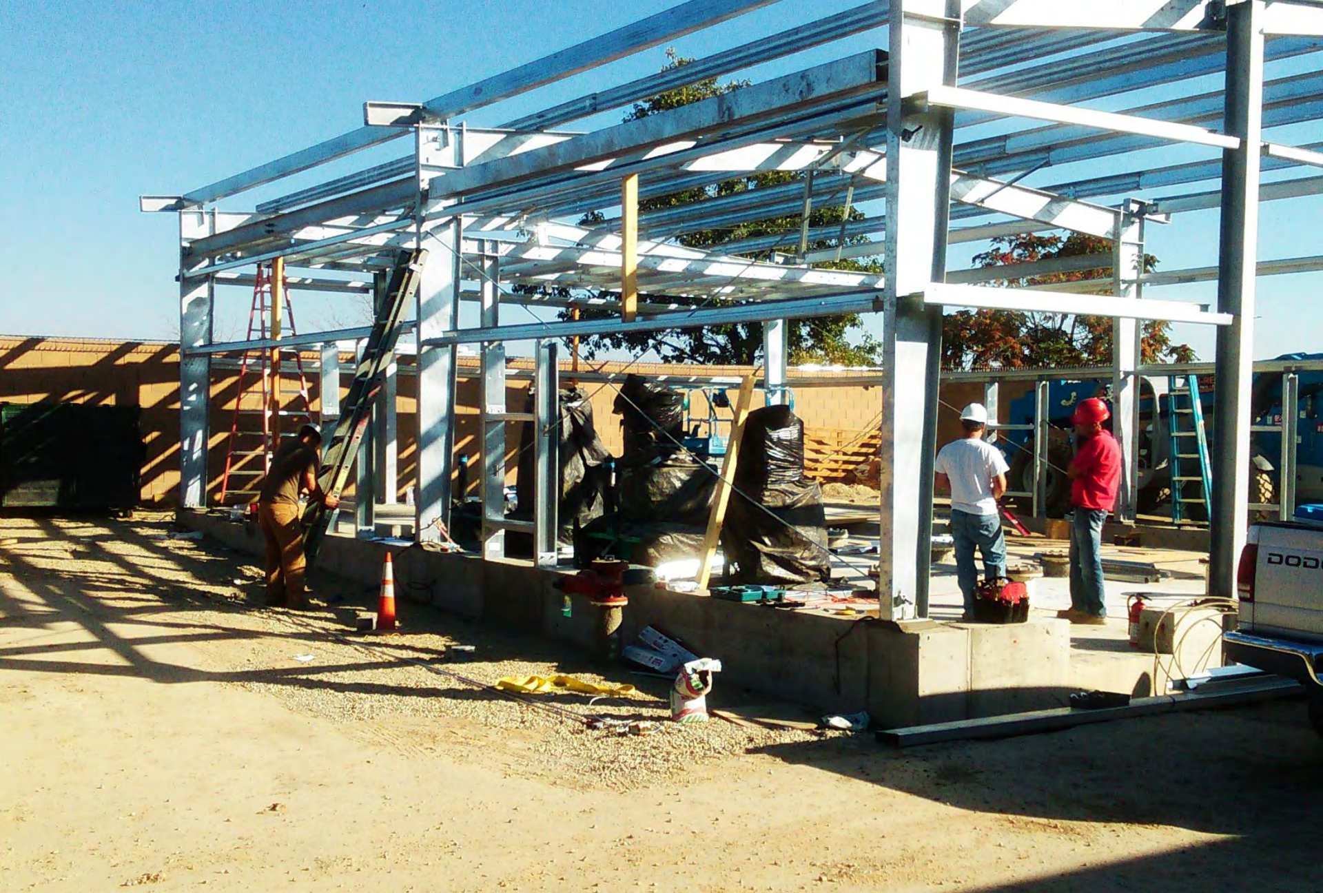
31AM Tie Rod bracing installed; note rod passing through ne
