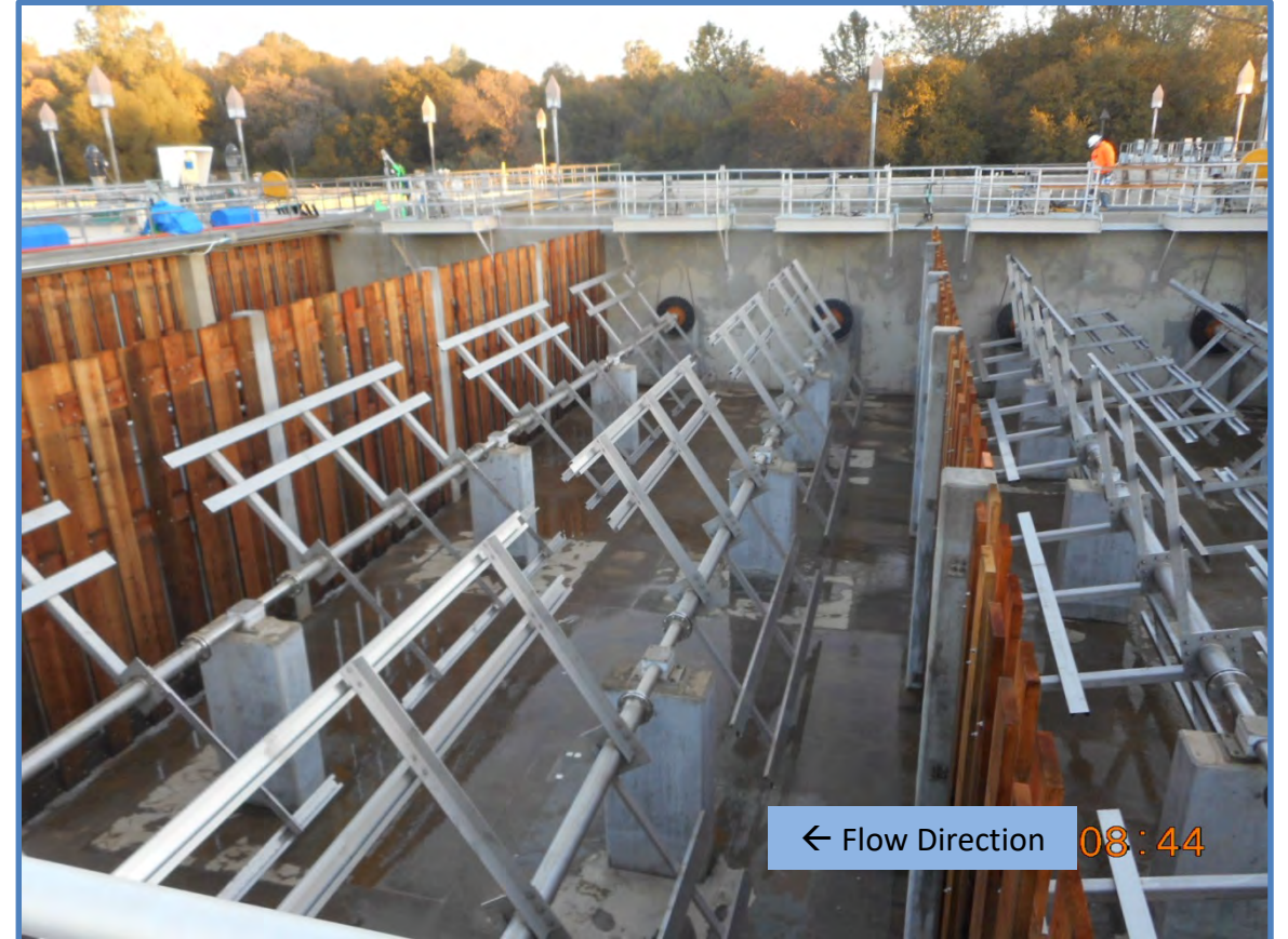
“AFTER” – More Effective Paddle-Wheel Flocculators
