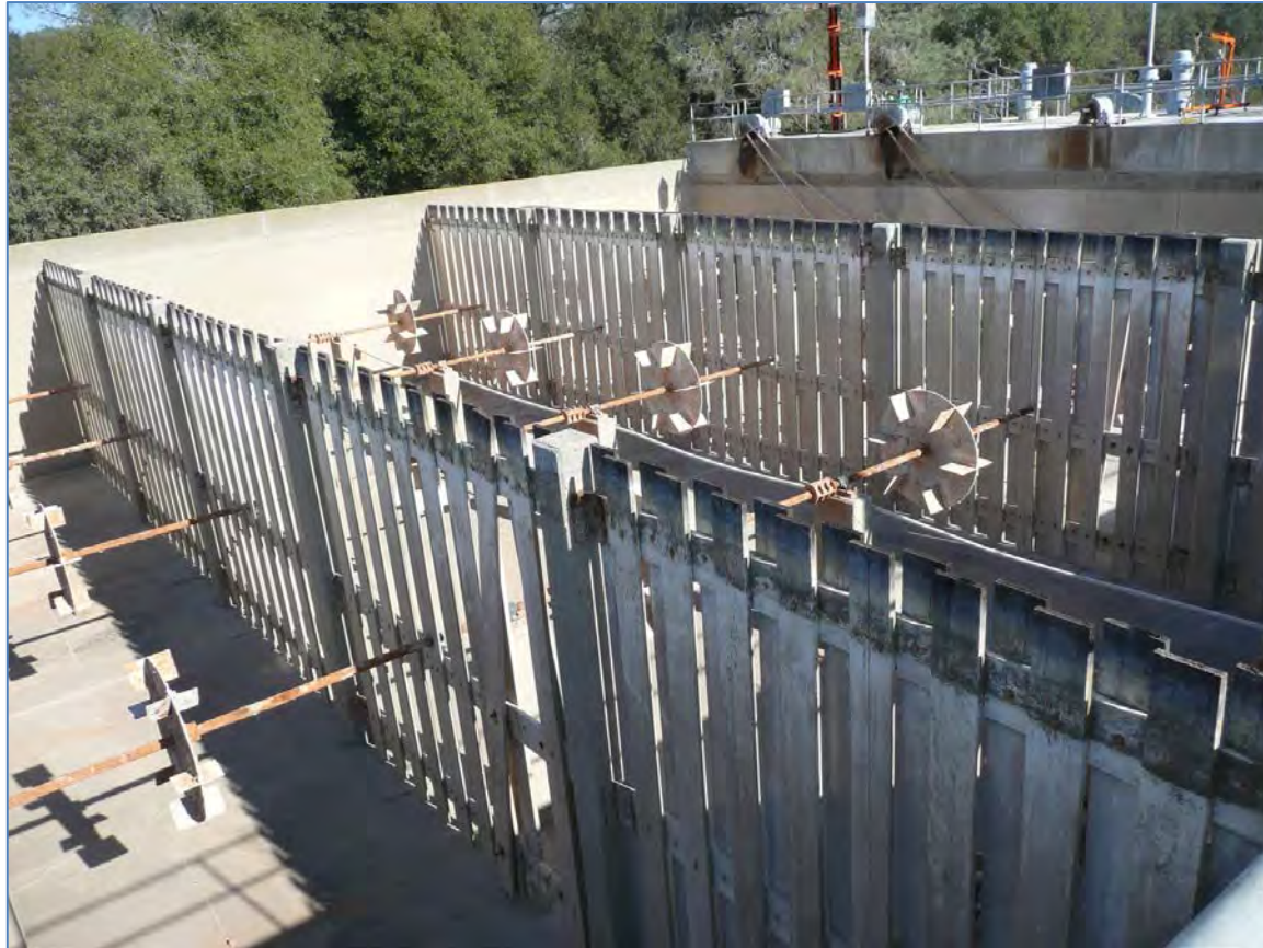
“BEFORE” – Existing (2) Redwood Baffle Walls
