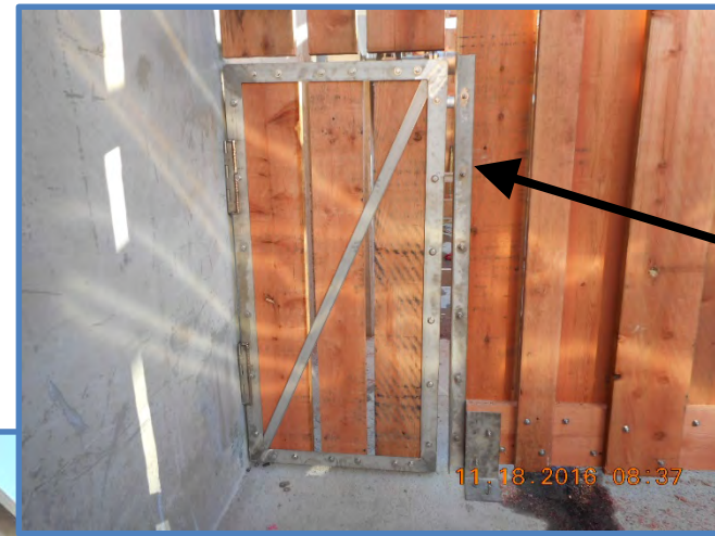
“AFTER” – Added Maintenance Access
