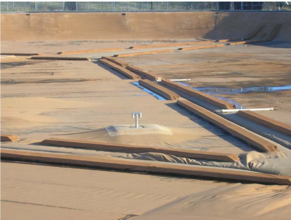
Figure 6. Photo showing the single “T” vent on the Kokila Cover.
