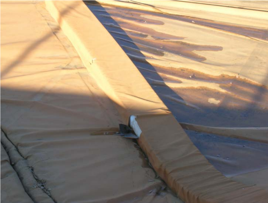
Figure 9. Photo showing damage to floats at side slope – North slope.
