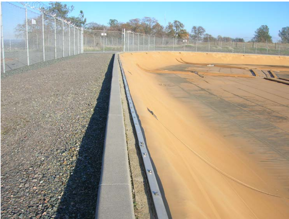
Figure 2. Photo showing typical condition of the perimeter attachment and concrete curb.
