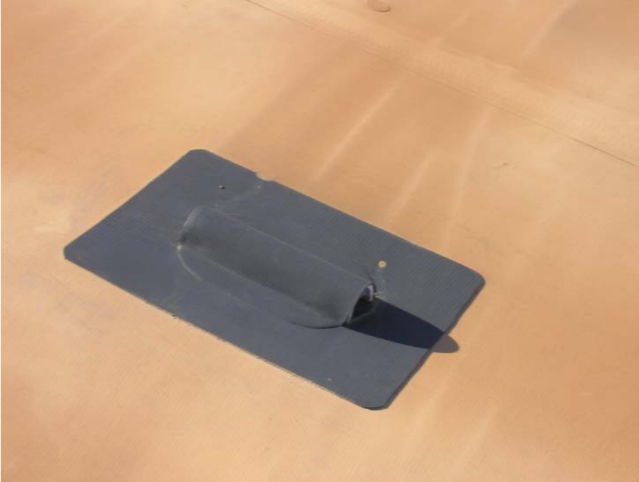
Figure 5. Photo showing typical prefabricated side slope air vent with ½ PVC tube and hole with screen under the tube.
