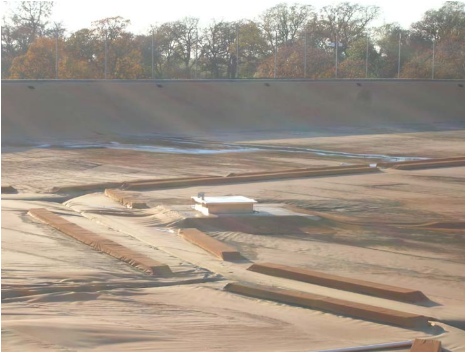
Figure 7. Photo showing the single 36 X 36 inch Hatch with vent and floatation System. Note distorted and wrinkled cover lower left of photo.
