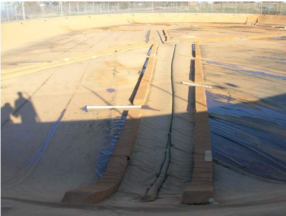
Figure 8. Photo illustrating distortion of floats due to steep side slopes and Lower water elevation. These areas are prone to damage due to stress.
