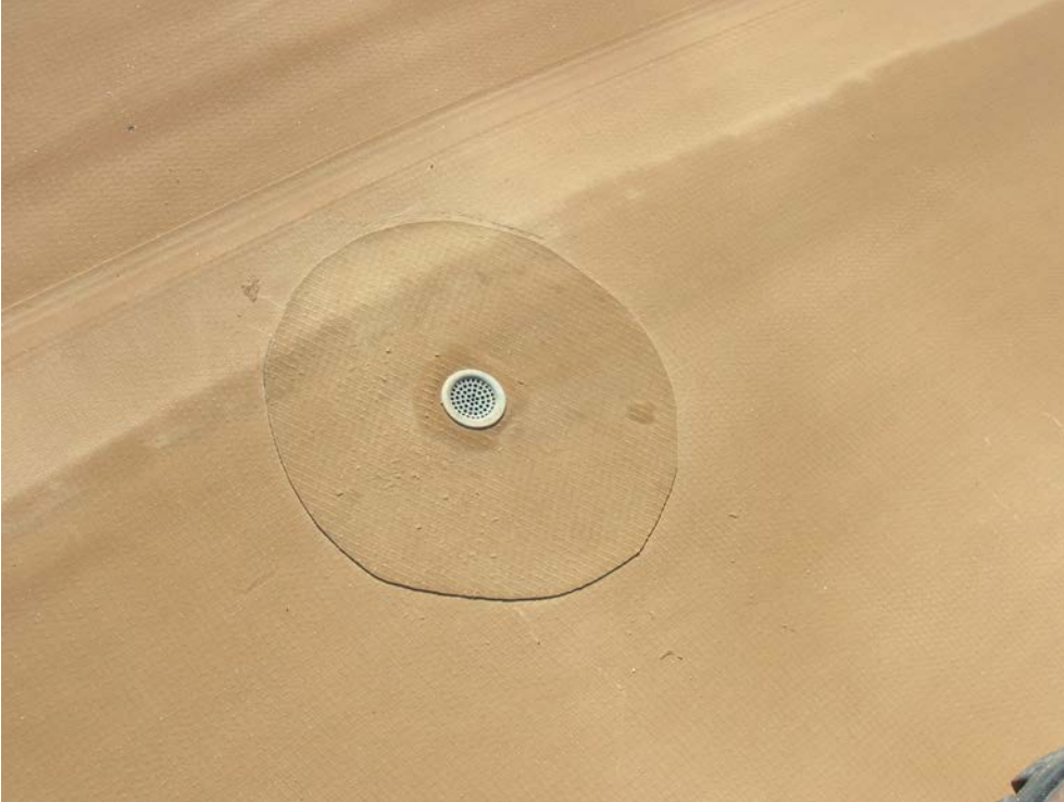
Figure 3. Photo showing typical current air vent detail with one-way valve.
